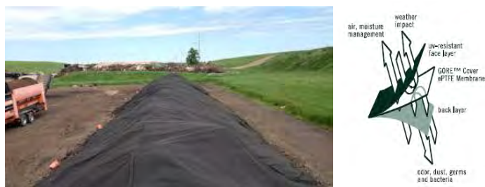
Figure 11. a) Membrane Covered Windrow, and b) Benefits of using Membrane (After GORE® Cover System-North America)
