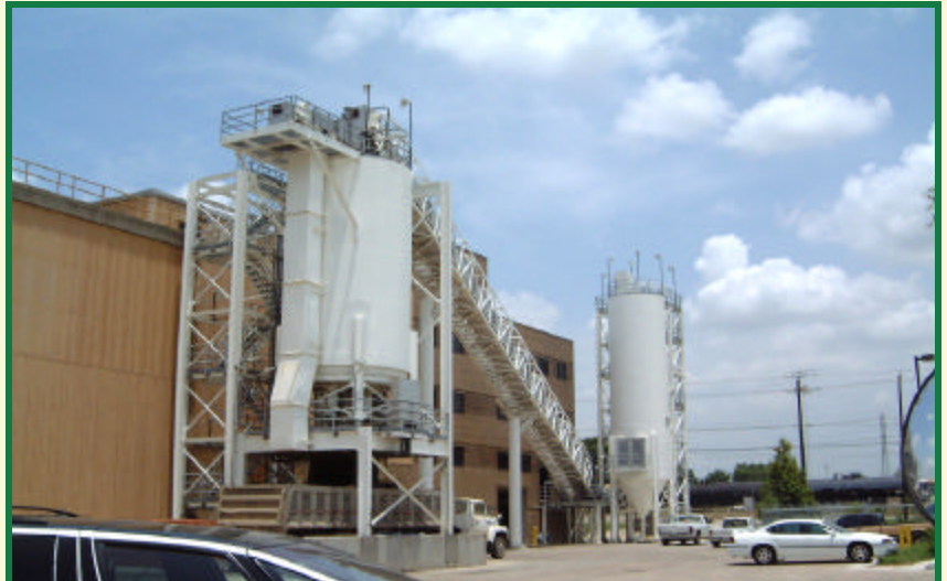
Lime Stabilization in use at a large metropolitan wastewater treatment facility
