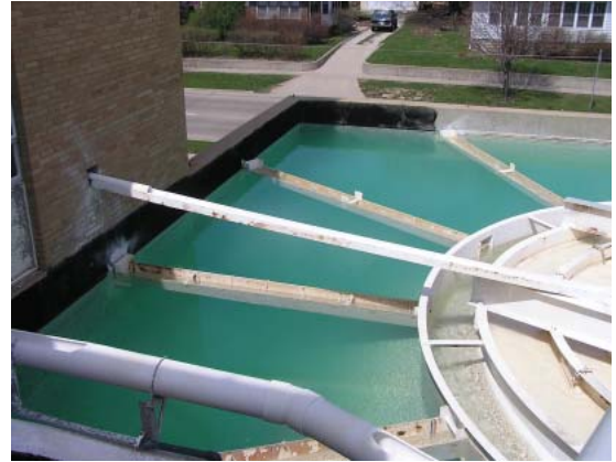
Above: Gravity flow from the Slurry Aging Tank to the softening basin is controlled by a Magnetic Flow Meter and a Pinch Valve.
