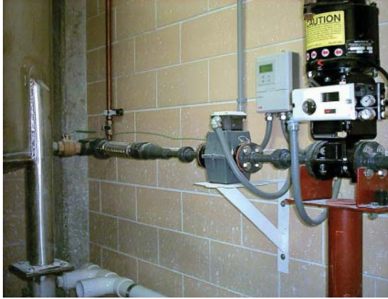
Above: Gravity flow from the Slurry Aging Tank to the softening basin is controlled by a Magnetic Flow Meter and a Pinch Valve.
