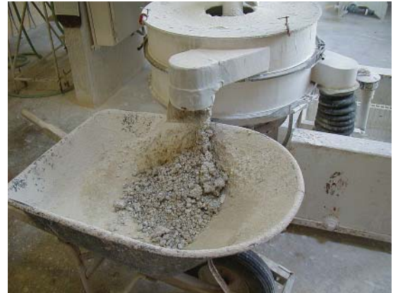
Above: Old vibrating screen shown discharging grit and lime paste.
