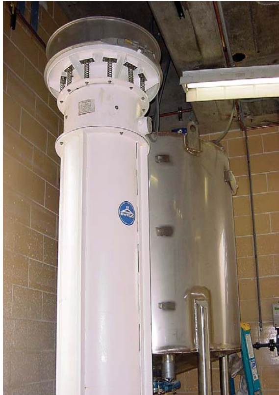
Above: Stainless steel vibrating screen installed above the Slurry Aging Tank to maintain gravity flow of the lime slurry from the discharge point of the lime slurry transfer pump.
