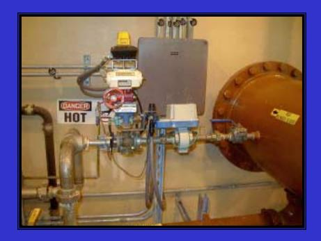
Lime Slurry is then added to the suction side of their Hidrostal Pump<sup>®</sup>. The Hidrostal Pump<sup>®</sup> then transfers the sludge/lime mixture into one of
