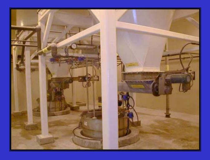
Each Slaker has a feed screw conveyor that conveys the lime into the Slaker in about 2 - 3 minutes per batch.
