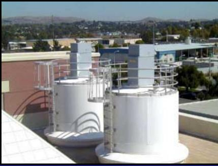
The System begins with unloading lime into one of two identical 45 ton Storage Silos.
