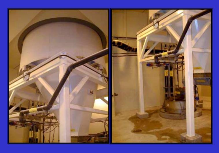
Each silo sits on four load cells and provides us with a very accurate quantity of tons of lime remaining in each silo.
