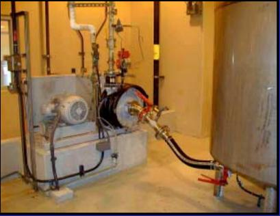
The Slakers protrude through the Slaking room floor and gravity discharge into the Slurry Aging Tanks. Each Slurry Aging Tank holds  $2^{1/2}$  batches of slaked lime. This allows the pumping loop system to operate continuously. Wemco Torque Flow® pumps are used for the Slurry Loop System.
