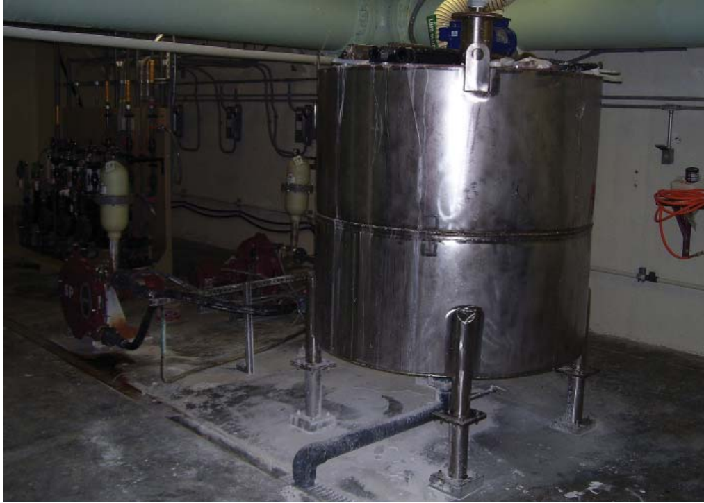
Above: Slurry Aging Tank holds 2-1/2 batches (500 gallons) of slaked lime for pumping by either Watson Marlow hose pump to the softening basin.
