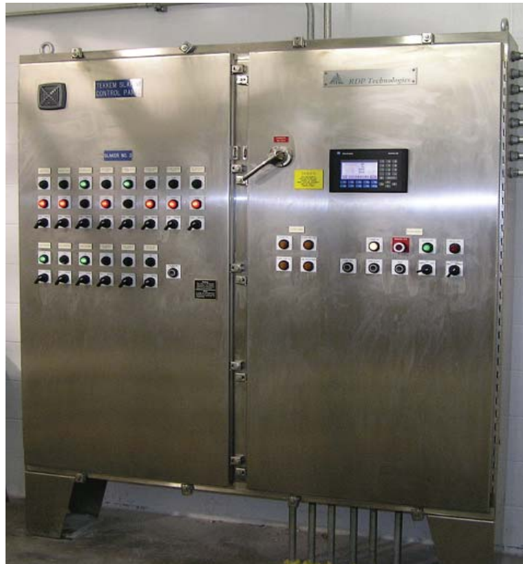
Left: Two Tekkem System Control Panels (one shown) each with an Allen-Bradley Panel View 550 control screen, which achieves complete system redundancy
