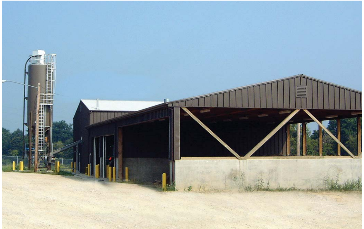
Above: Storage building in foreground and the Belt Filter Press/Pasteurization building in the background.
