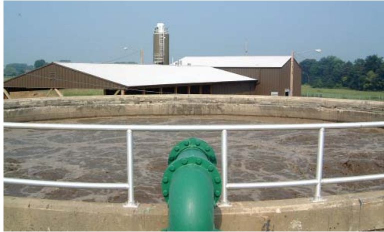
Above: The aerated sludge holding tank insures more consistent feed solids and “fresh” sludge to the Belt Filter Press.
