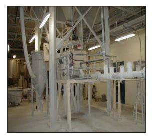
The new system included Bin Activators for each silo and Tekkem floor mounted 4,000 lb. per slakers. More efficient grit removal was accomplished using stainless steel circular vibrating screens. A Slurry Aging Tank was installed on the floor below
