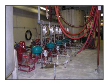
Lime slurry is pumped from one of two new Slurry Aging Tanks using double disc pumps. Each pump is dedicated to serving one of five softening basins
